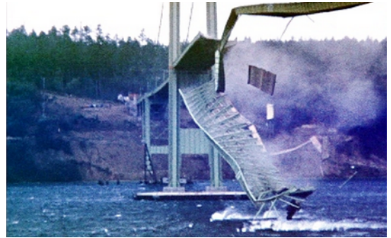
Figure 1: 1940 Tacoma Narrows Bridge failure
